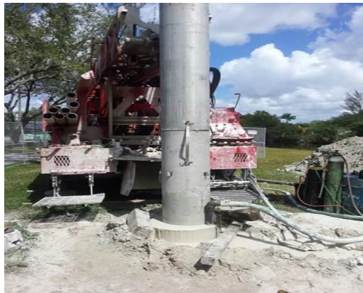
Well casing with centralizers
