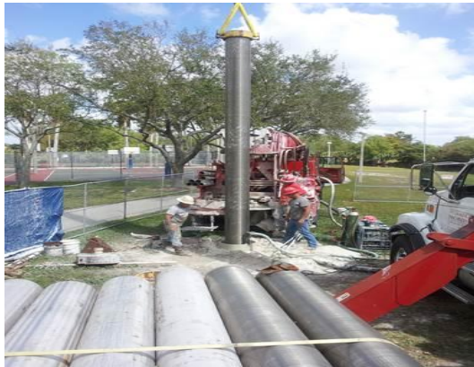
Installing the well screen
